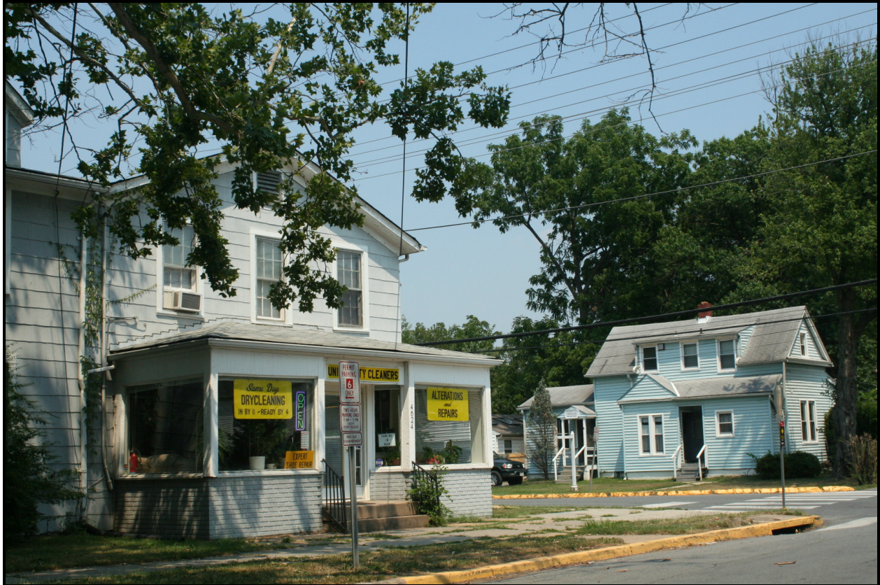
Looking northeast, Harrison Store/Trolley Stop Sweet Shop (PG: 66-021-11), 4622 College Avenue and 7501 Rhode Island Avenue ( EHT Traceries , 2007)
